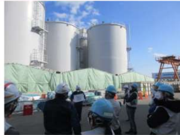
K4 tank area
