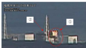
Picture of explosion at FDNPP unit 3*
