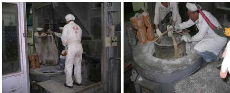
圖二、熔銅用石墨坩堝爐體築爐作業
