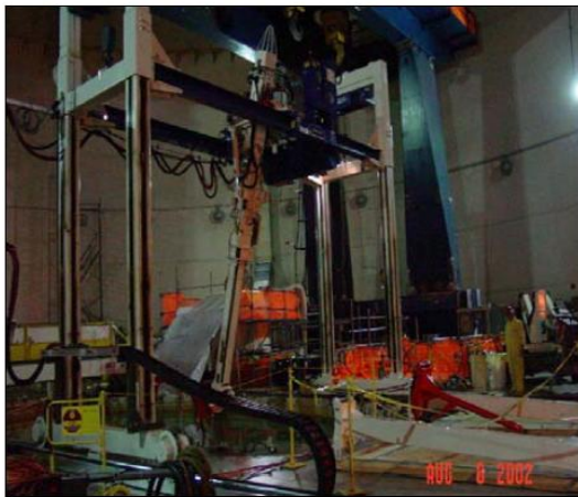
Grant Machine Structural Assembly
