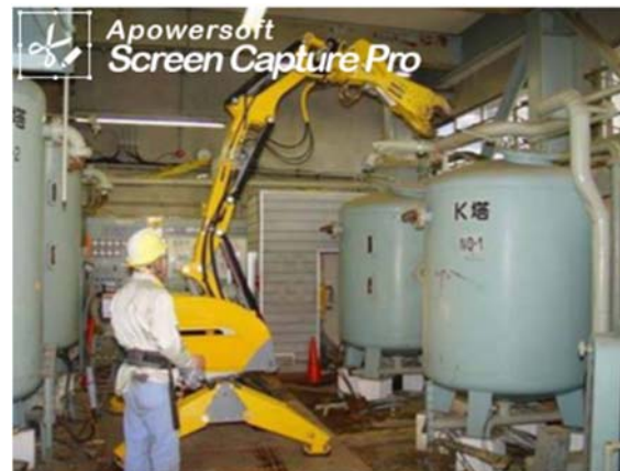
(b) Brokk 180 unit cutting pipes with steel shears in Japan
