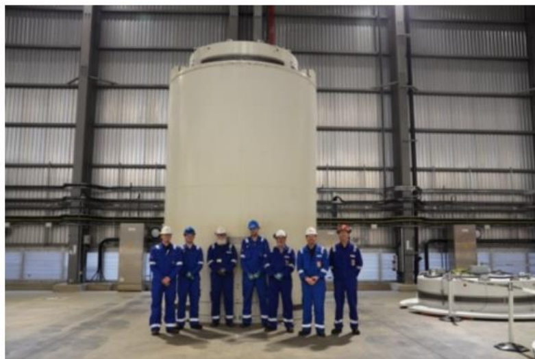
The HI-STORM MIC cask in place in the Sizewell B store (Image: Holtec)
