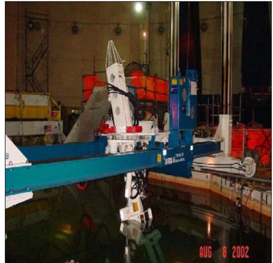
Cavity Vacuuming With Grant Machine
