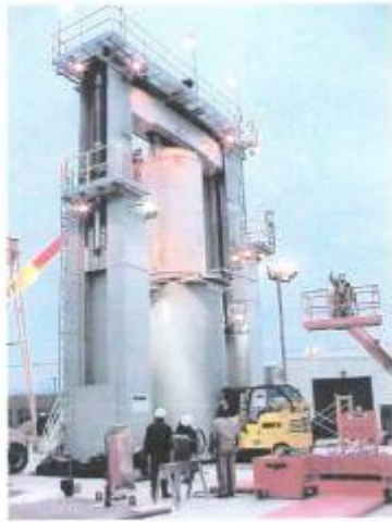
Dresden Cask Transfer Facility - Completed
