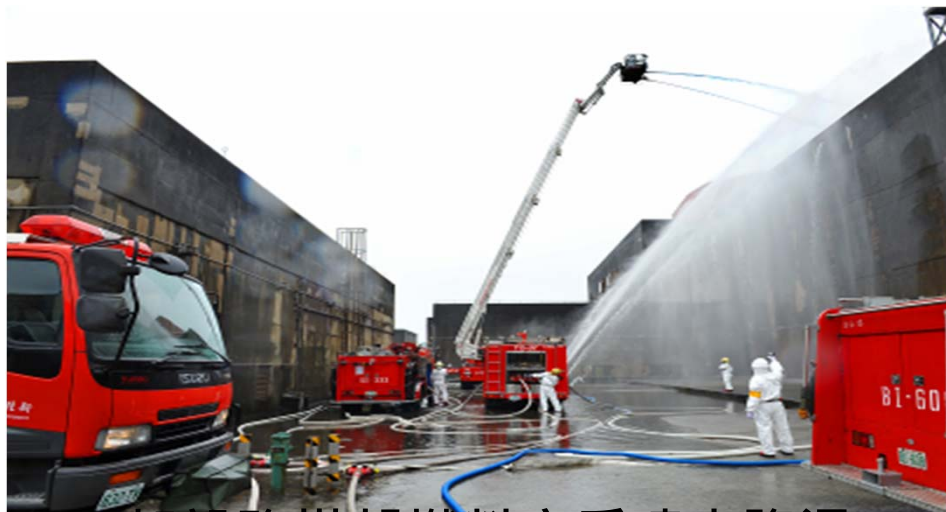
架設砲塔朝燃料廠房噴水降溫
