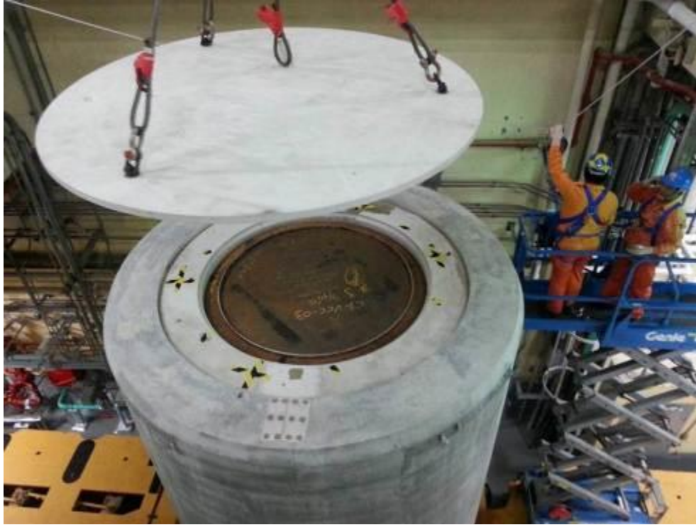
(a) VCC 頂蓋吊至#1 RB 5F 暫貯
