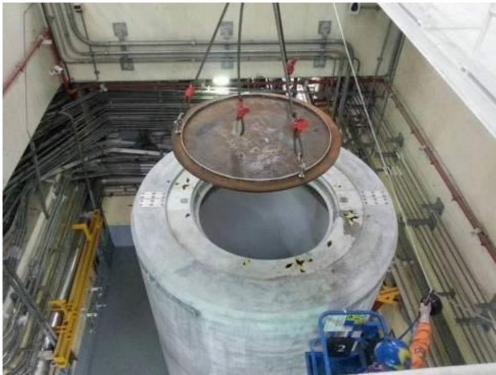
(b) VCC 屏蔽塞吊至#1 RB 5F 暫貯
