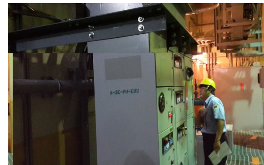
Inspection on 480V MCC in MS NPP
