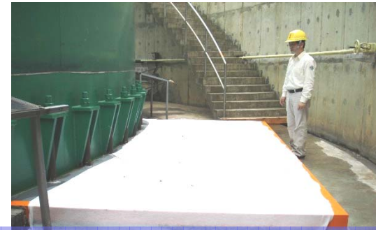
Inspection on reinforcement of EDG fuel oil storage tank in CS NPP
