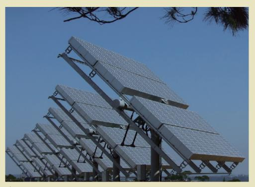
↑Ground Mounted 5 kW HCPV System
