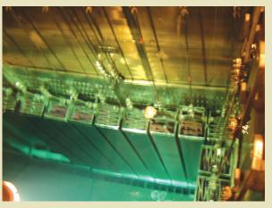
↑ The Container Loaded with Compressed CRB Blades Hanged Inside the Spent Fuel Pool
