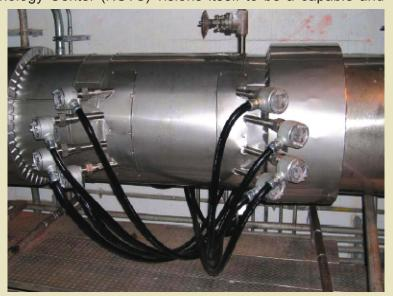
↑The UFM system (Caldon LEFM CheckPlus) installed at Kuosheng NPP
