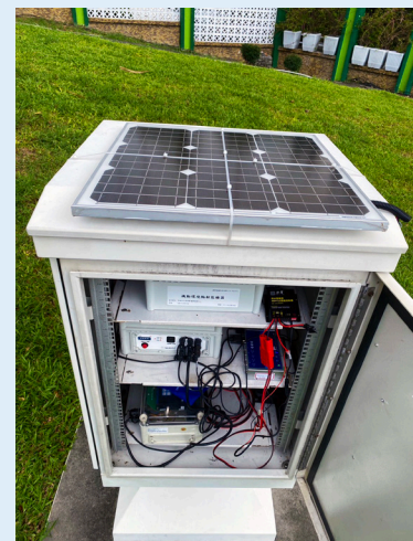
▲ Expansion of Monitoring Station Power Supply with Solar Charging Module
