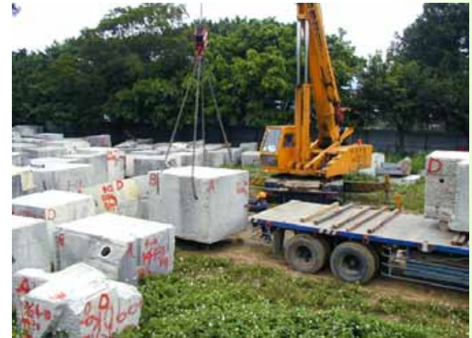
Dismantled Concrete Block Preparing for Storage
