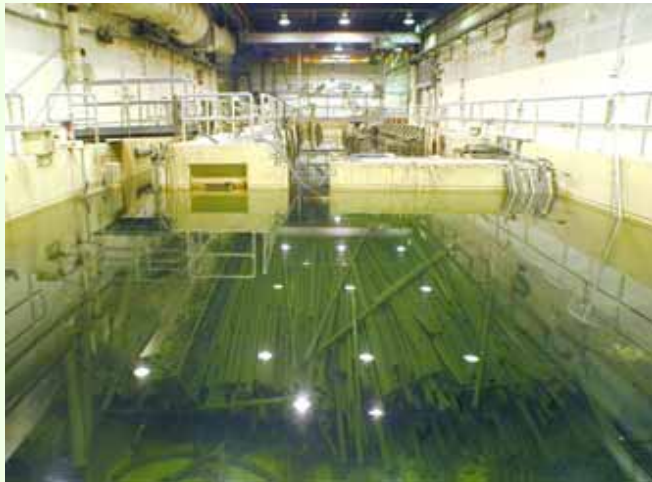
Aluminum Tube Inside the Spent Fuel Pool
