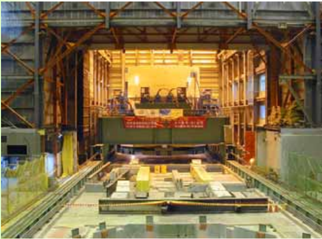
TRR Reactor Shielding Block Removal
