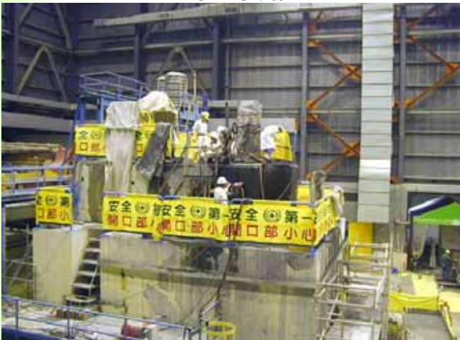
TRR Reactor Shielding Block Removal
