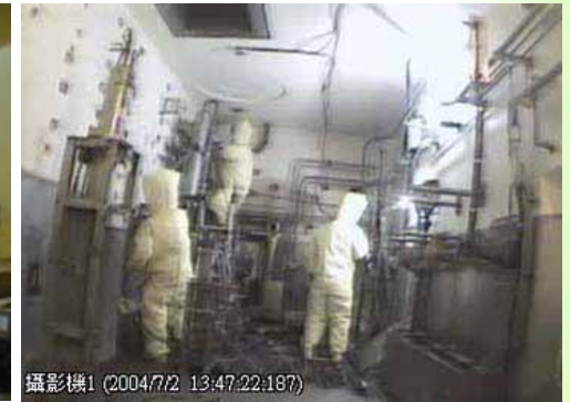
Equipments Inside Hot Cell Dismantled
