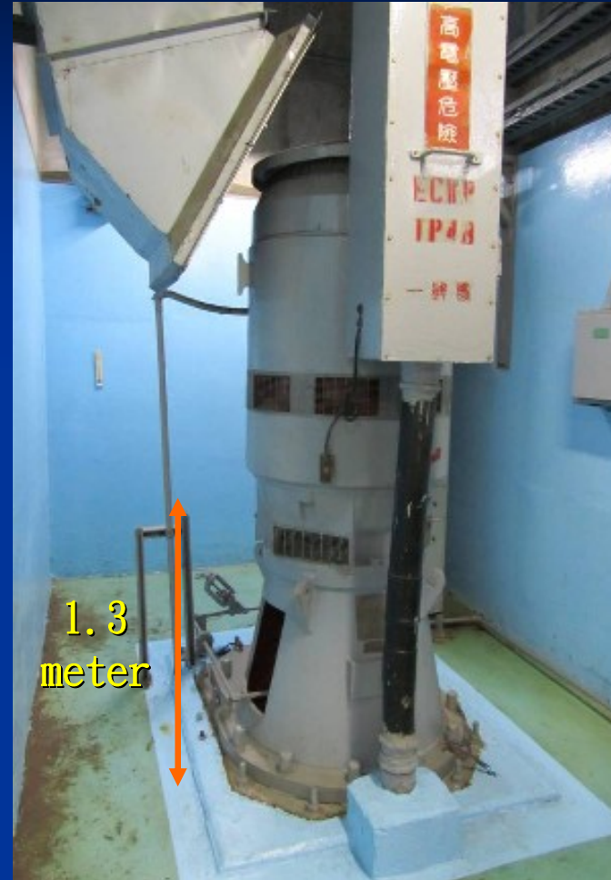
ECW motor 7.9 meter above mean sea level
