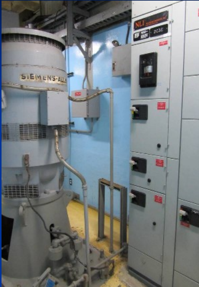
ECW pump and motor (Floor El. 6.6 meter)
