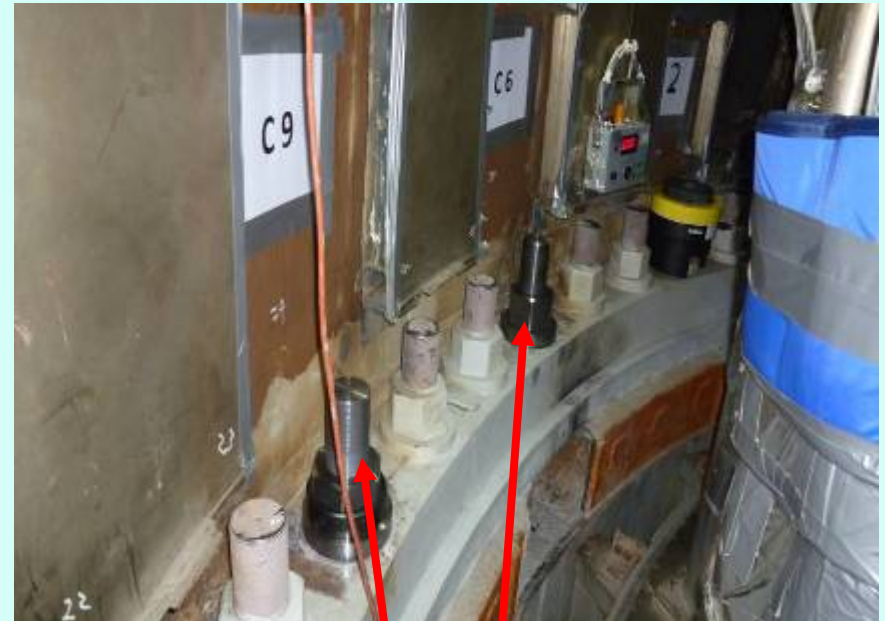
New studs after installation
