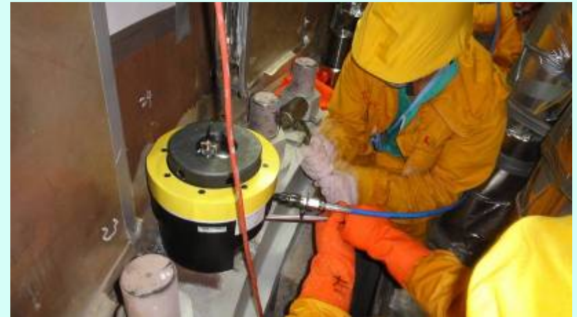
Installation and Preload
