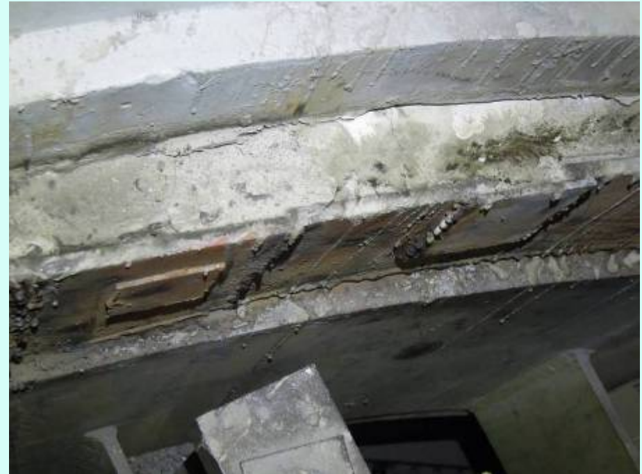
Recovery of the surrounding concrete
