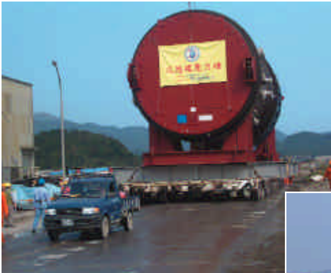
Figure 6 RPV transport process
