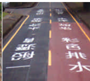
Figure 56 Road paved with quenched slag
