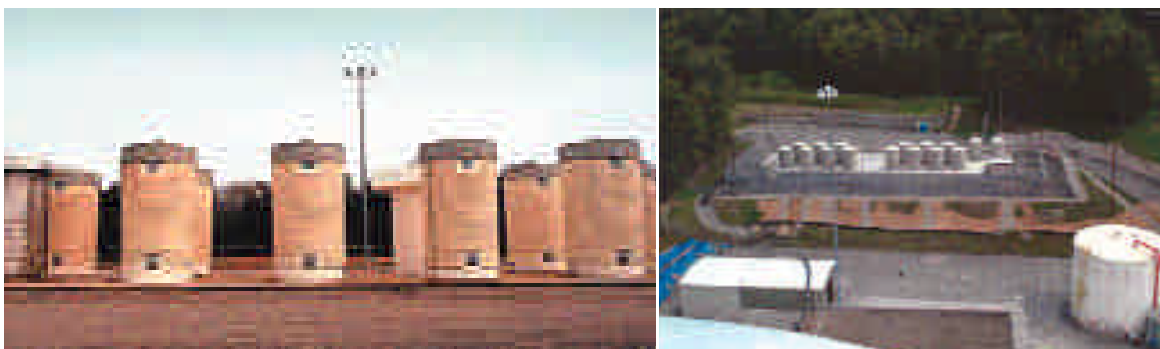
Figure 70 A concrete cask storage facility for spent nuclear fuel at the Yankee Rowe NPP in U.S.A.
