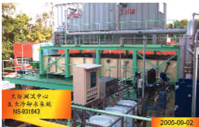
Figure 52 Primary/secondary cooling systems for the high-power torch
