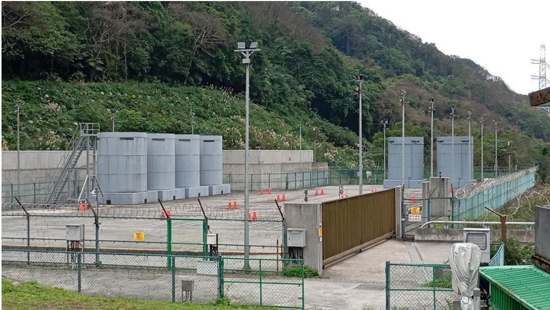
Figure D-1. Spent Fuel Outdoor Dry Storage Facility of Chinshan NPP
