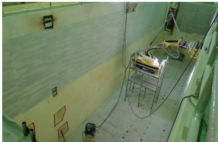
TRR燃料池池體除污 Decontamination of spent fuel pool surface of the TRR
