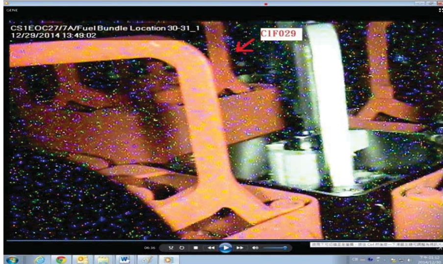
Figure 2. Raised fuel channel (in the background) in comparison to a fresh fuel assembly.
